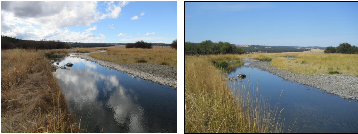
Figure 8. Photo point collected for the Lower Camas Creek site 2007 (right) a year after levee removal looking downstream with the lowest two J-hook structures visible. During 2018 (left) looking downstream from the middle of the reach where the lowest two J-hook structures are visible.
